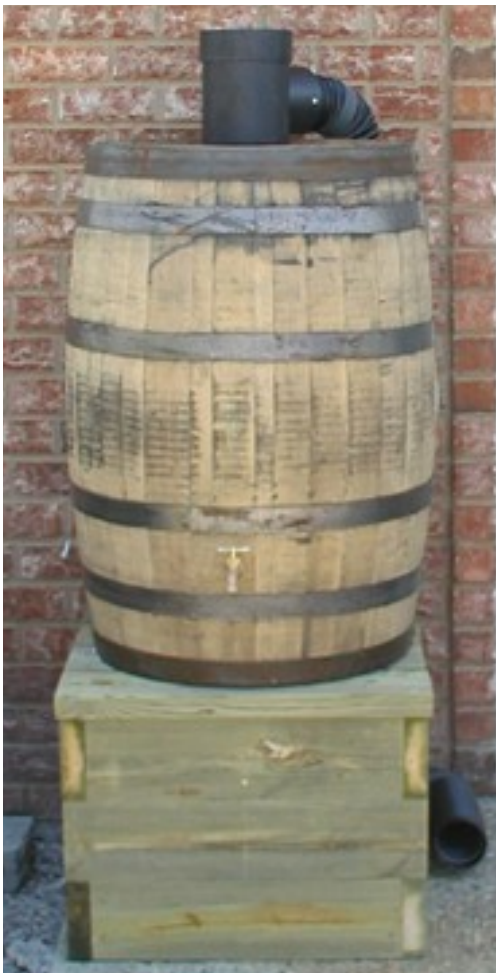
A newly constructed wooden rainbarrel sits atop a custom-built wooden stand.
